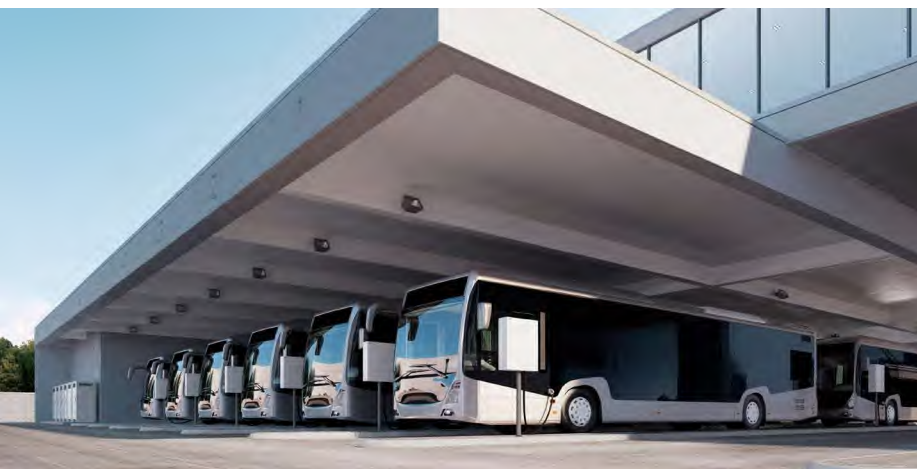
— HVC Depot Boxes and power cabinets, lined up at a depot site.
